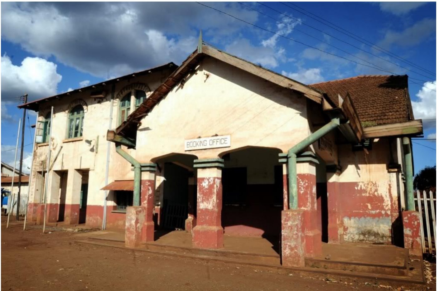
Another depressing view of Moshi Railway Station (Recent)
